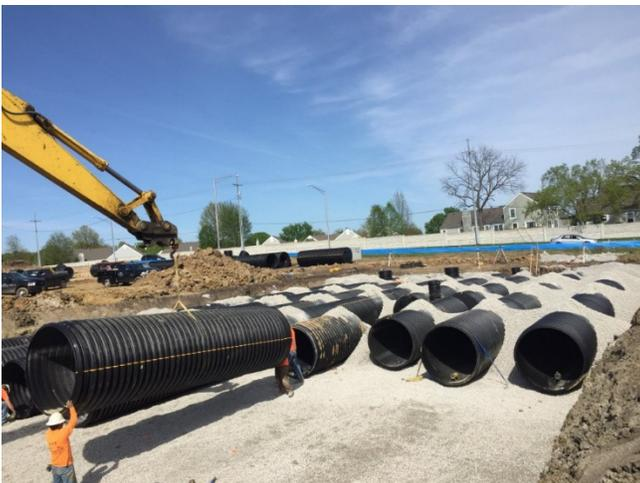
The large diameter HDPE pipe was offered as an alternative instead of CMP because it allowed easier coupling options, product functionality, and would not require any on-site alterations. Additionally, typical soil-tight CMP couplers utilize nuts and bolts to fasten the joint while HDPE pipe connections use a gasketed connection in the bell and spigot water tight joints. The manifold tees and 90 degree elbows were also easy to assemble onsite with Prinsco's GOLDLOCK Couplers.
